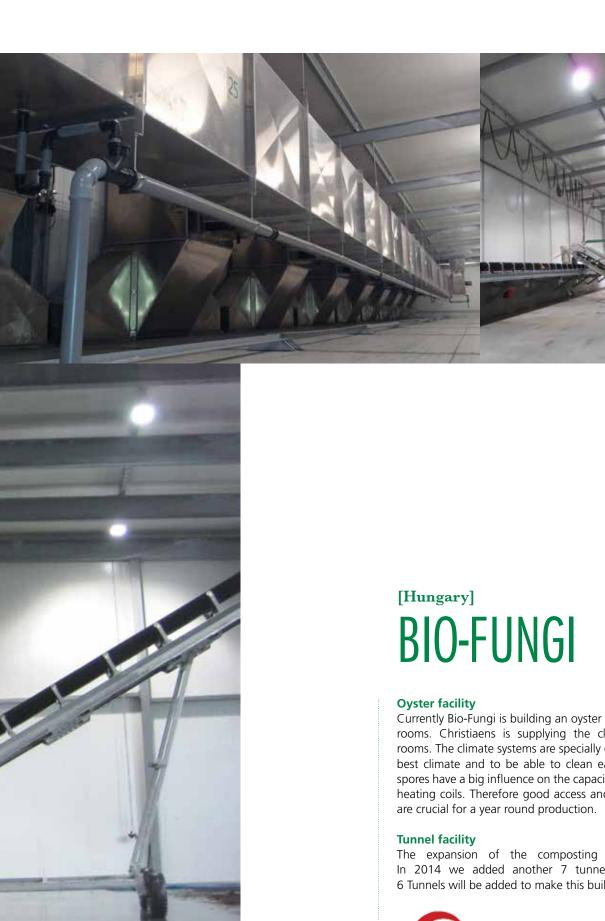
Currently Bio-Fungi is building an oyster farm with 12 growing rooms. Christiaens is supplying the climatisation for these rooms. The climate systems are specially designed to create the best climate and to be able to clean easely. Besides hygiene spores have a big influence on the capacities of the cooling and heating coils. Therefore good access and cleaning possibilities
